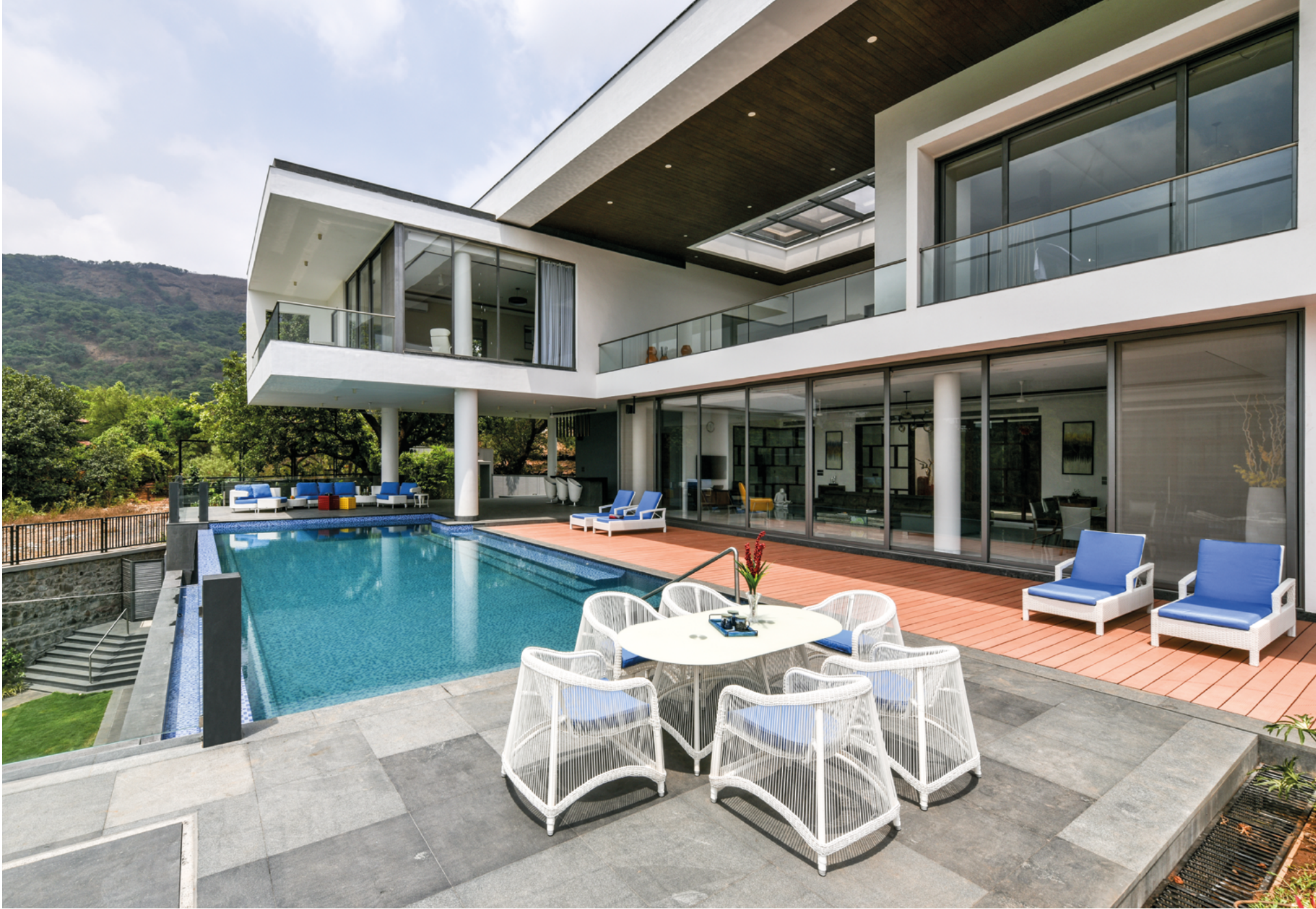
Heavy weather: Concrete and brick were the main construction materials, while large overhangs form decks as well as providing protection from storms and heat
